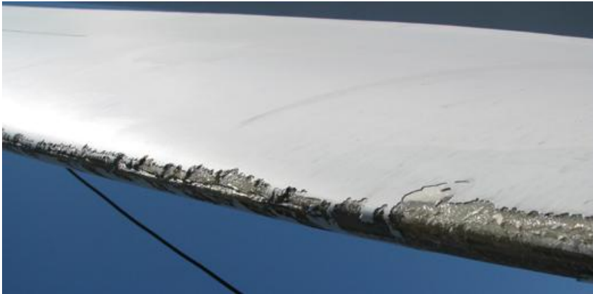
Example Edge Erosion Before Repair
