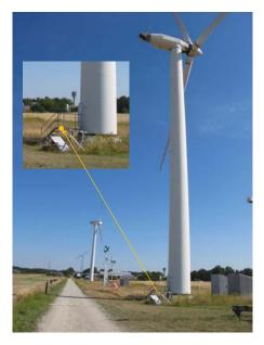
Figure 5: Photo of the NordTank wind turbine used during the measurement campaign. The use point used as a reference for the TST is presented in a zoomed frame. Behind the wind turbine one the short-range WindScanners (R2D1) can be seen.
